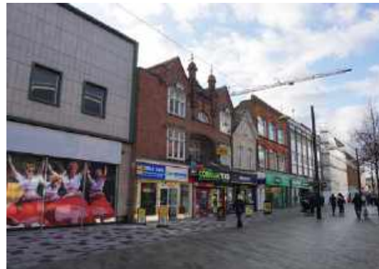
Fine grain buildings on the south side of High Street
